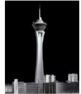
Las Vegas Tower Acceptance Paul Balfe AFIAP FAPS
